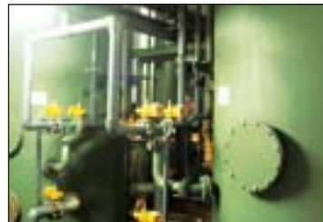
Steel de-iron filter (N093-T01)
