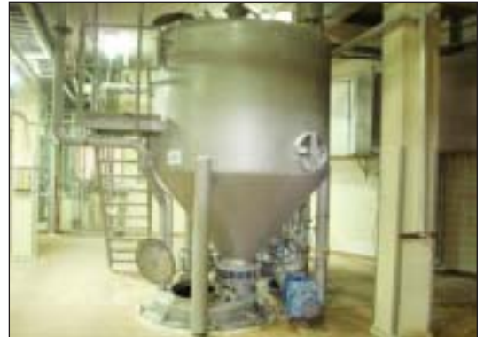
Ss dough tank (22-5-33), ymf: 1997, with pump, pneum. stop valves
