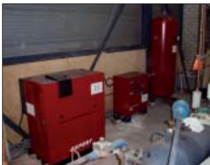
Expert schroefcompressor/droger en buffertank Expert screw compressor/dryer and buffer tank
